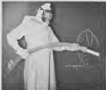
This sandblasting job requires Domingo J. Werlema of Mechanical-Shops to wear this Fresh Air Hose Mask in addition to other protective clothing.
